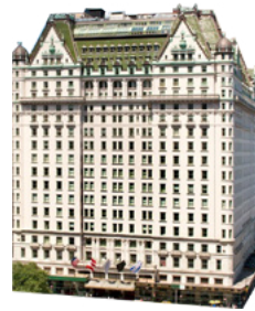
The Plaza 1 Central Park South
