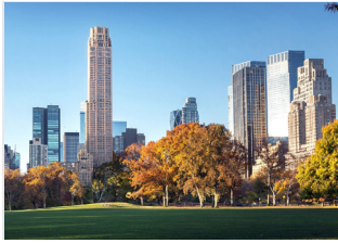
220 Central Park South
